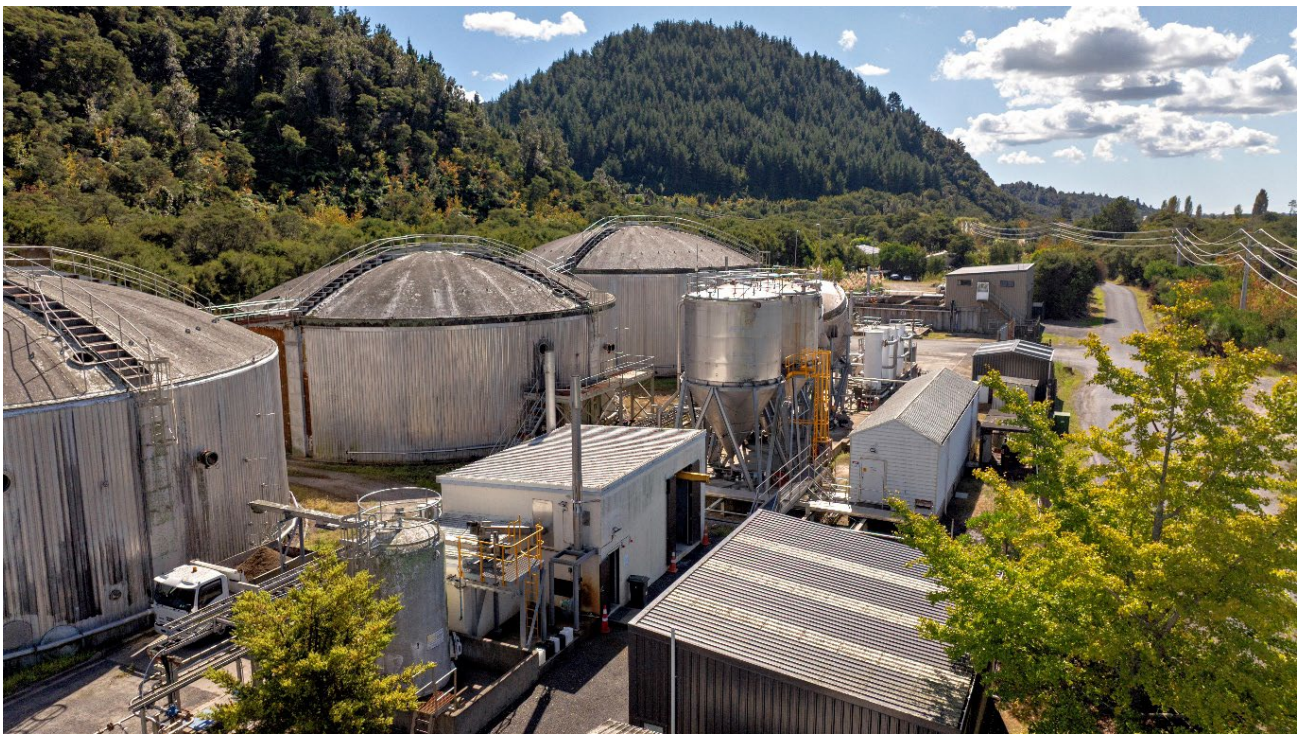
Wastewater Treatment Plant in Kawerau.
