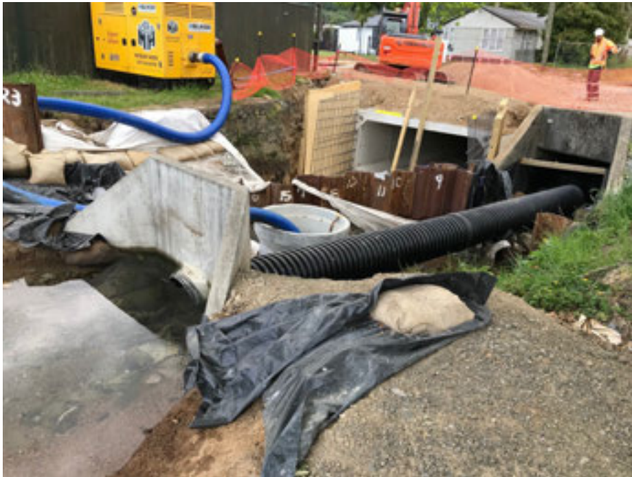
ABOVE: Culverts replaced on River Road provide additional capacity in extreme weather events.
