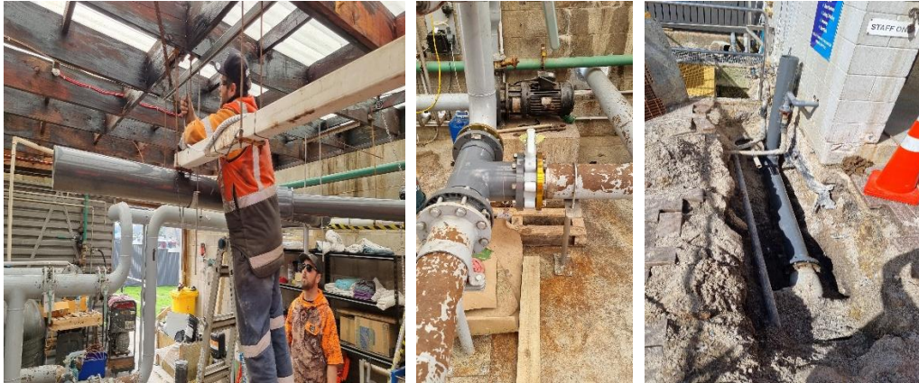
Figure 5: SPA Pool Leak Repairs
