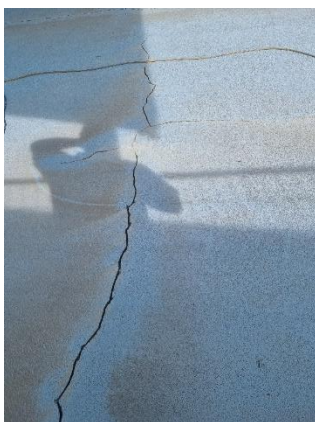
Figures 3: Cracks in main pool walls
