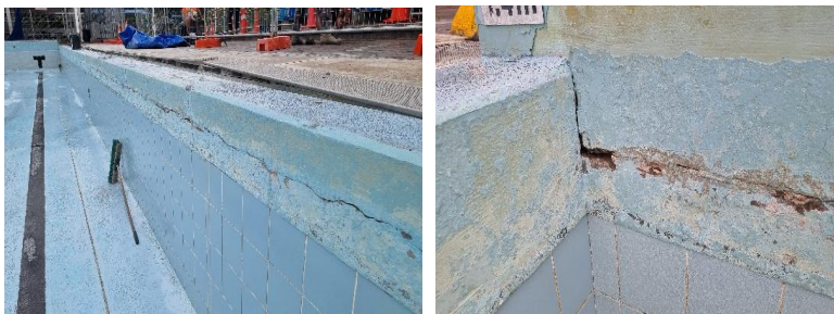
Figures 3: Cracks in main pool walls
