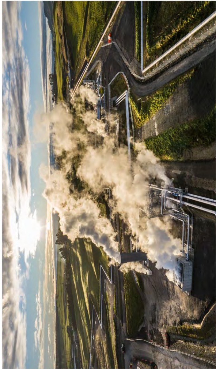
Figure 4: The Te Huka power station steaming ahead, currently piloting the reinjection of non-condensable gases (primarily CO 2 ) back into the geothermal reservoir (image supplied by Contact Energy)
