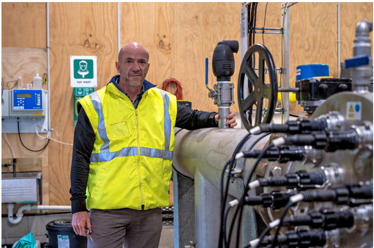
Group Manager Operations and Service Riaan Nel at the Water Treatment Plant following the installation of four new pumps to provide greater resilience and more efficiency in the provision of drinking water to the community.
