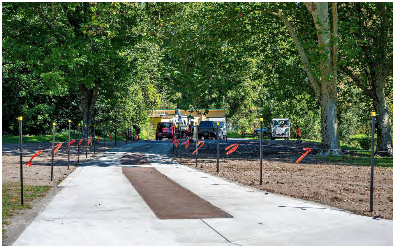
Improved access to the River Road drinking water taps for the community and staff into the Water Treatment Plant on River Road.
