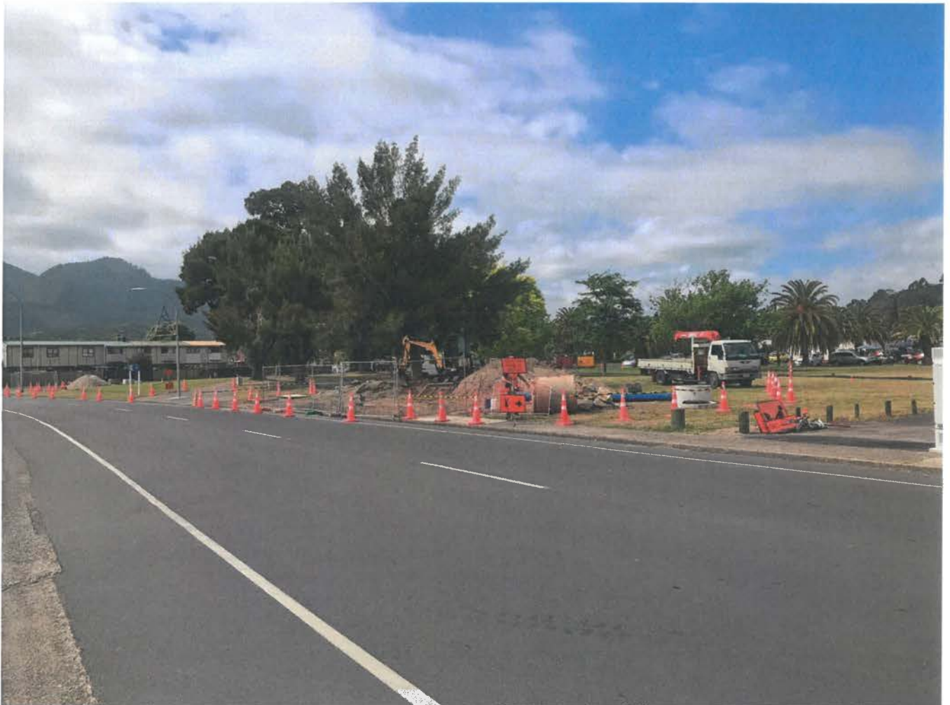
PIPEWORK RENEWAL ALONG PLUNKET STREET
