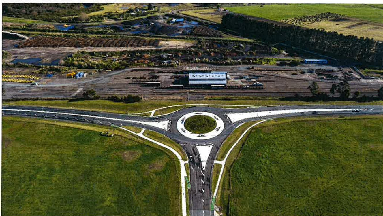
The roundabout on State Highway 2 developed for entry into the Pūtauaki Trust Industrial land.
