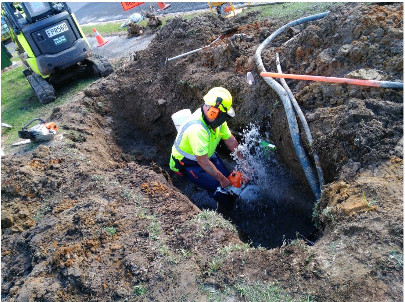
Kawerau's drinking water reticulation (pipe) replacement project.
