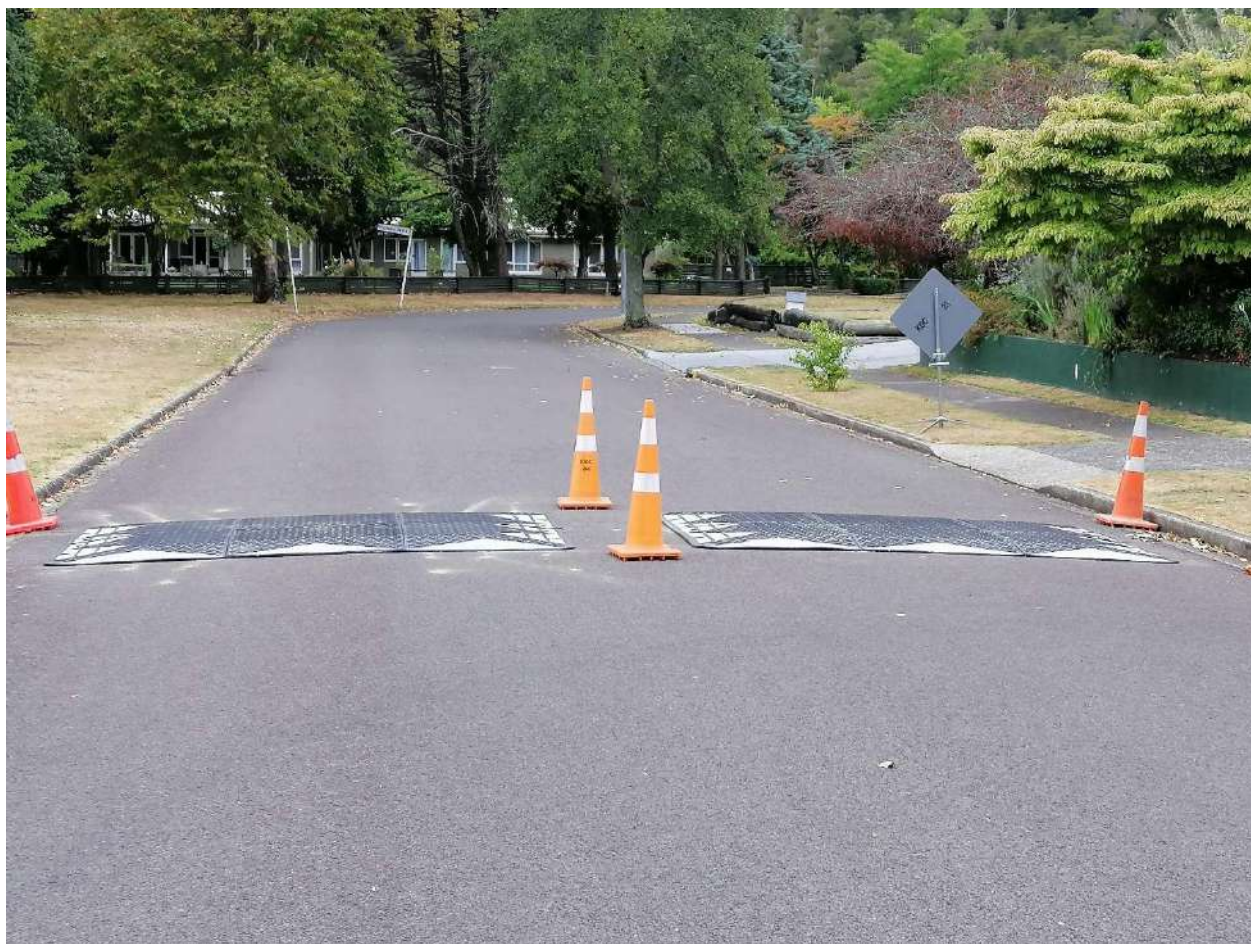
SPEED HUMPS INSTALLED ON MASSEY STREET
