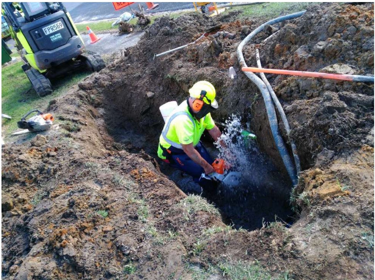
STAFF WORKING ON WATER PIPE
