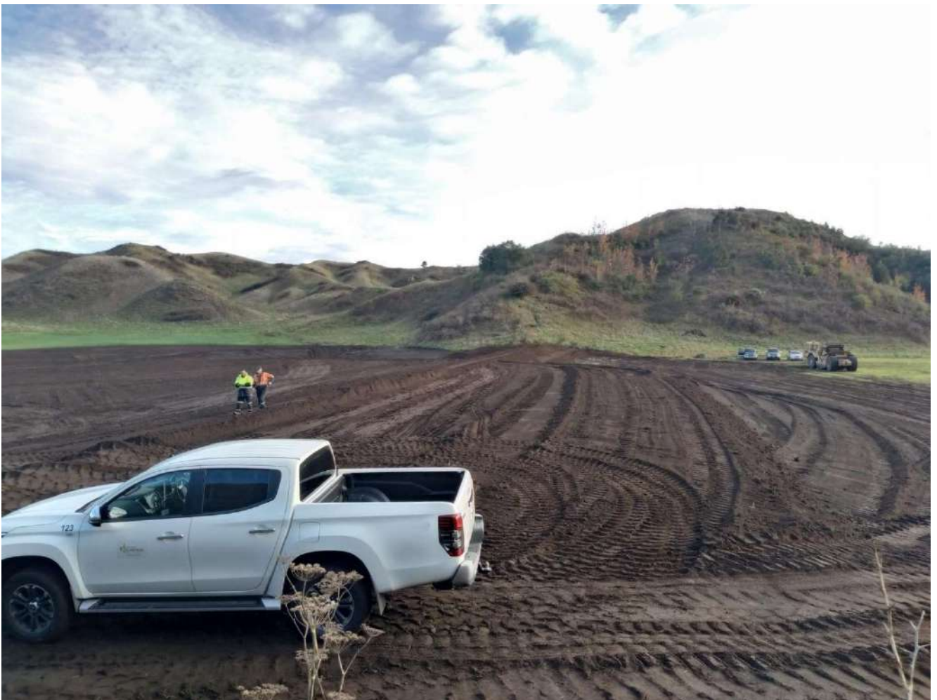
WORK ON STORMWATER DETENTION BASINS, AT HARDIE AVE
